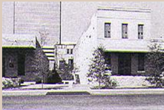
Warehouses fronting on Fourth Street.
